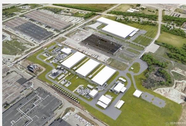
New York Hub Design (under construction)
